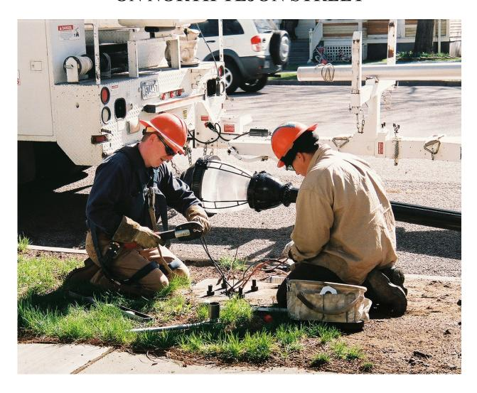
**PREPARING TO HOOK UP THE WIRES:** With the old aluminum pole removed and safely stored on the truck trailer, the two-person crew from Colorado Springs City Utilities made the necessary adjustments to the wiring. Note the helmeted globe of the new historic streetlight visible between the two workers.
