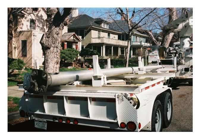
IT'S "BYE-BYE" TO THE MODERN POLE: The old aluminum streetlight pole, 30-feet high, was taken down and placed on the truck trailer to be hauled away. It will be recycled to a new location, probably on a major street where the pole's extra height and modernity will be appropriate.
