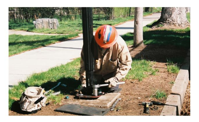
**BOLT IT DOWN:** The worker on the ground used a socket wrench to quickly bolt the new historic streetlight firmly into place on the old streetlight base.
