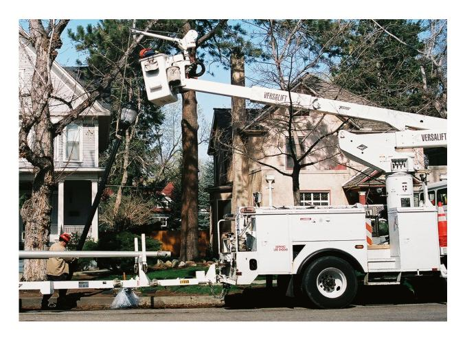
**ALMOST THERE:** As the new historic streetlight became progressively airborne, the worker on the ground began to move the bottom of the streetlight pole into position over the electrified base of the light.
